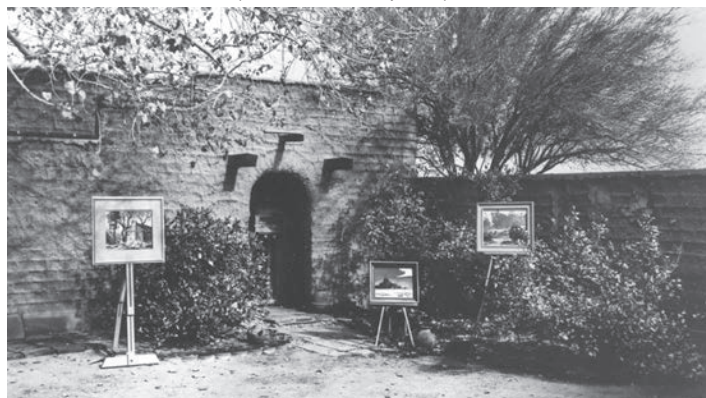
The Charlton adobe served as the Guild's gallery 1956-1963. Designed by Gerald W. Charlton in 1933-34, it was home to his widow, artist Irene Zimmers Charlton, until her death in 1997. It is now "Irene's Adobe" and part of 29 Palms Inn, down the street from today's 29 Palms Art Gallery.
